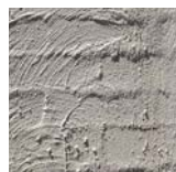
Bagged Brickwork
