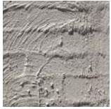
Bagged Brickwork
